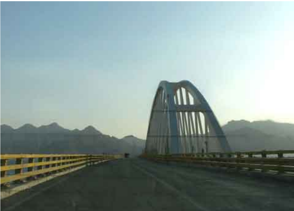
The causeway and bridge built across Lake Urmia was completed in November 2008. There is concern that it inhibits circulation within the lake and may exacerbate environmental issues caused by the lower water levels. Photo Source: Wikipedia
